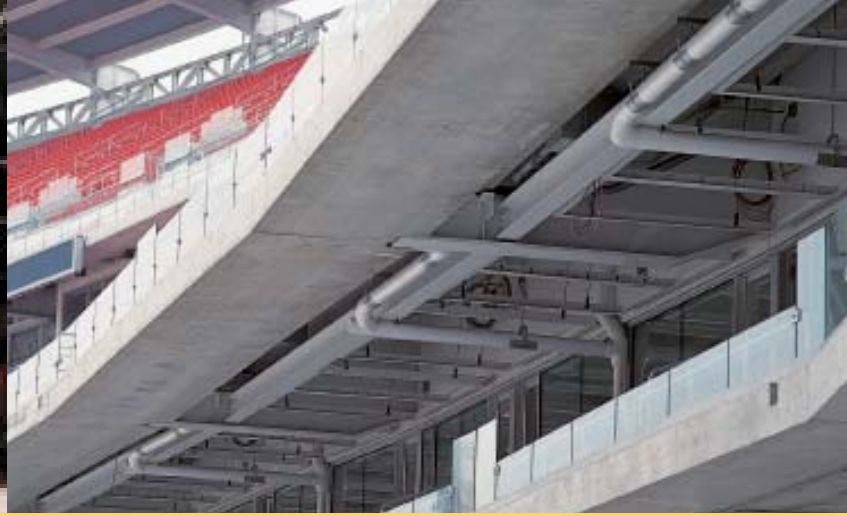
Most chilled water supply and return lines (left) were insulated at a 1" thickness; outdoor lines received 2"-thick insulation and were heat-traced. Roof drains (right) were insulated with 1"-thick 1000°F Pipe Insulation from Knauf and covered with white PVC jacketing to provide weather protection and a more attractive finished appearance.
