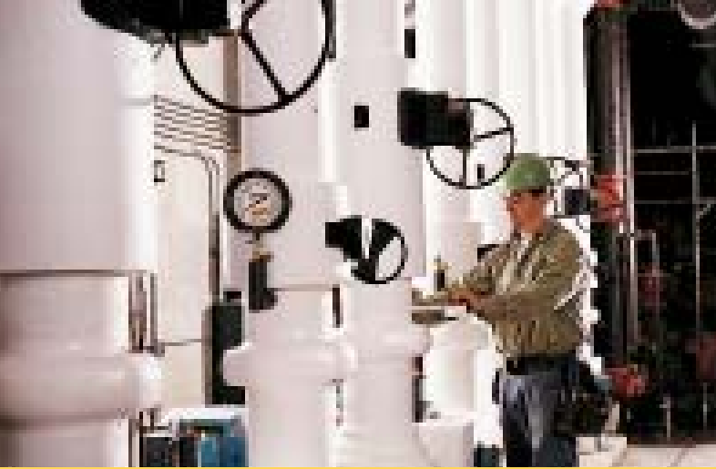
Most chilled water supply and return lines (left) were insulated at a 1" thickness; outdoor lines received 2"-thick insulation and were heat-traced. Roof drains (right) were insulated with 1"-thick 1000°F Pipe Insulation from Knauf and covered with white PVC jacketing to provide weather protection and a more attractive finished appearance.
