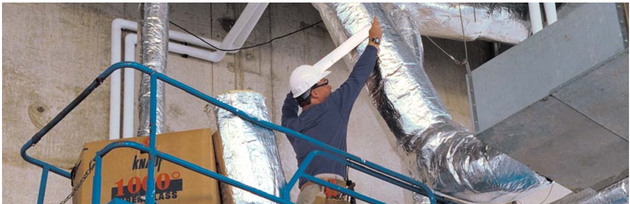
Knauf Duct Wrap is used to insulate supply ducts servicing upper-level courtrooms.
