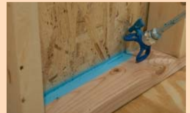
EcoSeal spray sealant should be sprayed on all joints, gaps and horizontal seams prior to insulation.
