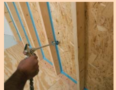
EcoSeal dries in a few hours, making it possible to insulate the same day as application.
