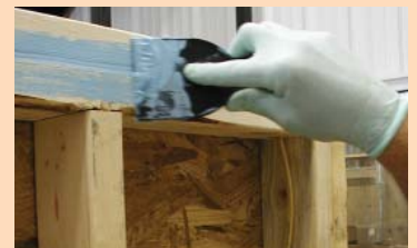
EcoSeal also coats the face of gaps smaller than 1/8", like the joint of double plates, shown, effectively sealing the joint.
