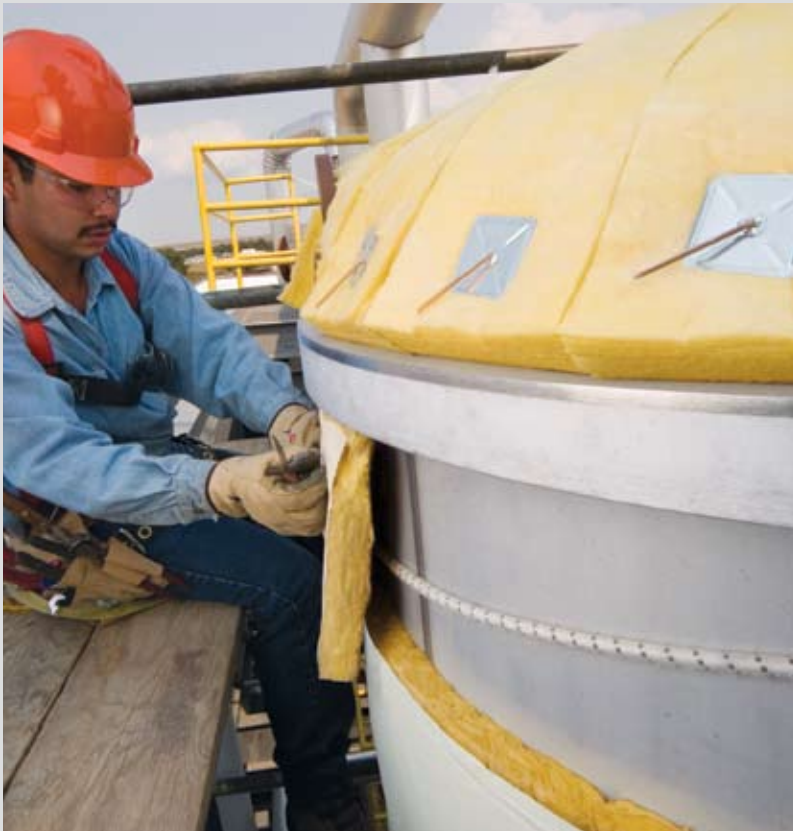
Knauf KwikFlex offers flexibility and compressive strength in a blanket form.
