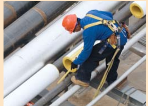
Knauf's "mandrel-wound" forming process prevents gaps and inconsistent densities, making notch out sections easy and clean.
