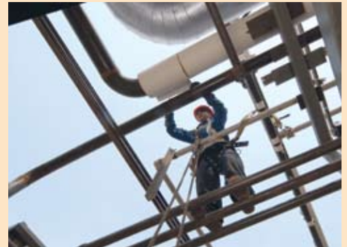
The pressure sensitive self-sealing lap eliminates a need for staples, additional material and tools.
